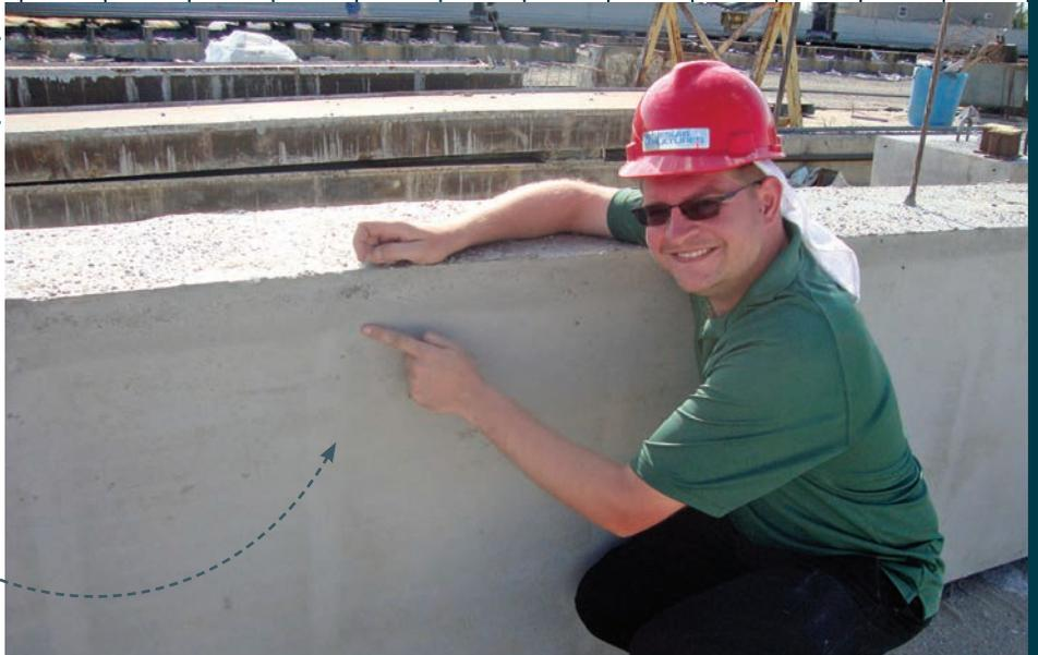
Feys works with Coreslab Structures in Marshall, Mo., which has made 30-foot beams and 60-foot beams for the project. In a February test, they poured a 60-foot beam. “It went good, but not perfect,” Feys says. “It seems like the 60-foot flow distance is a step too far.”
