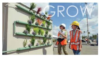
Wall of Plants The gravity-fed, vertical garden uses filtered greywater to feed the plants.
